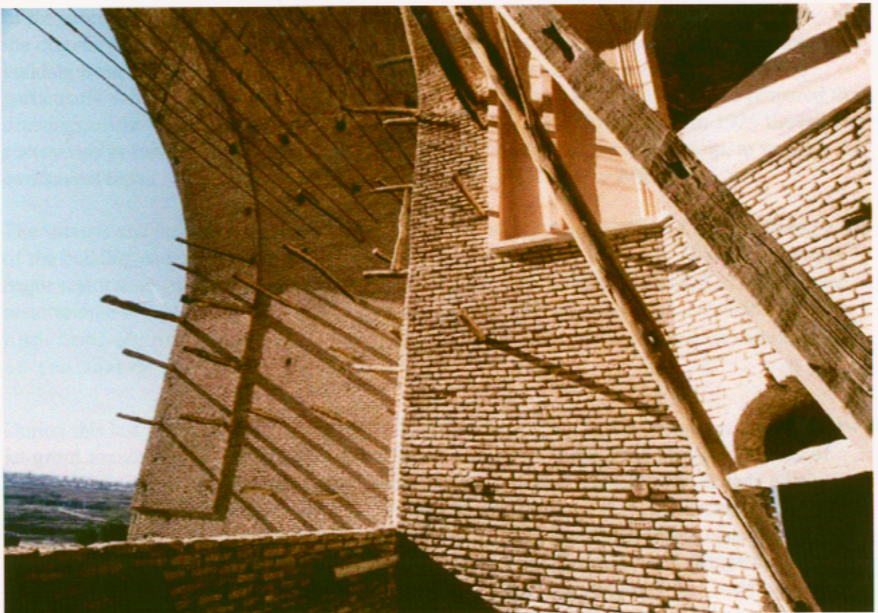
Scaffolding putlogs in the main portal arch
