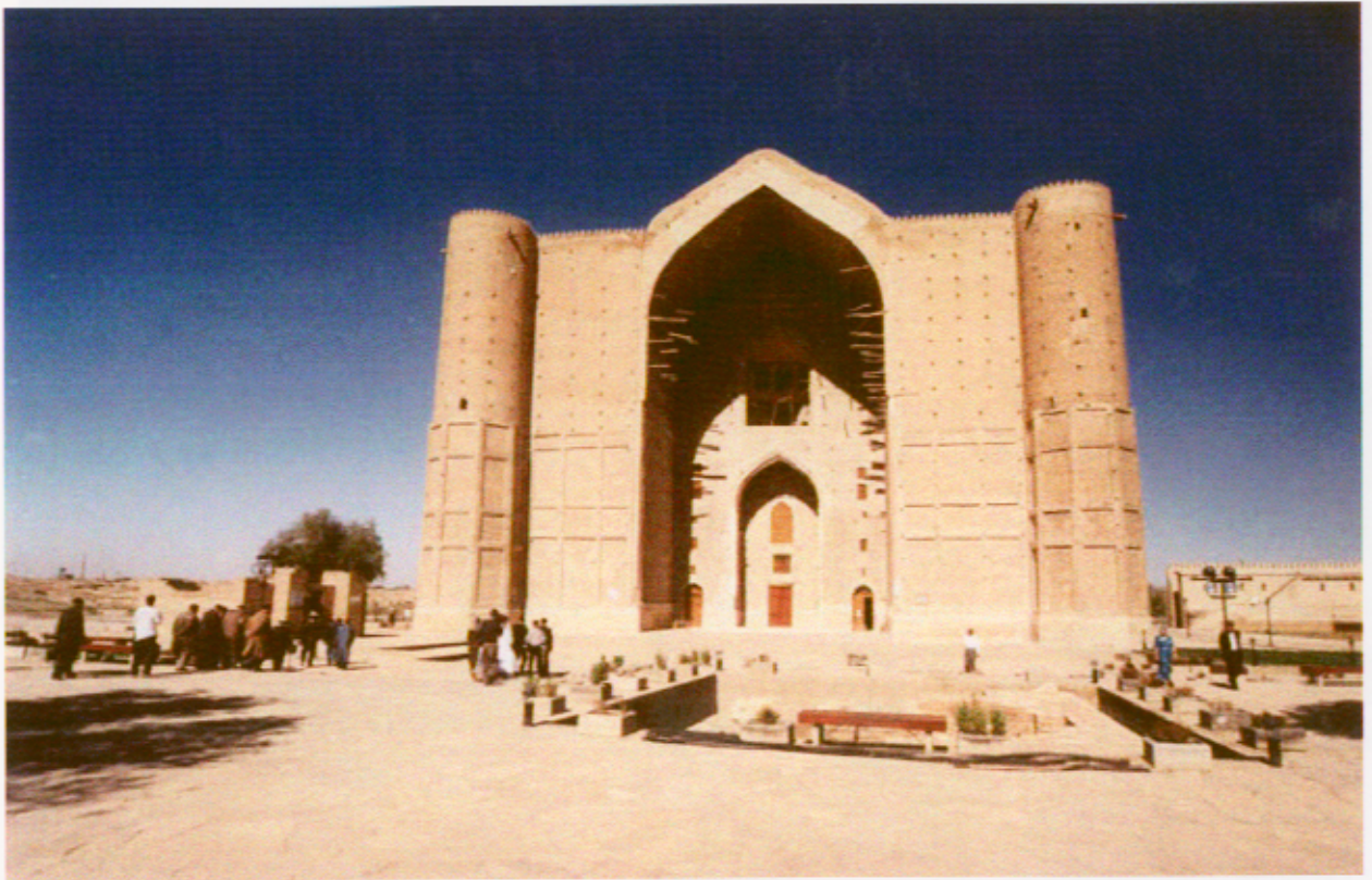
South front (main portal)
