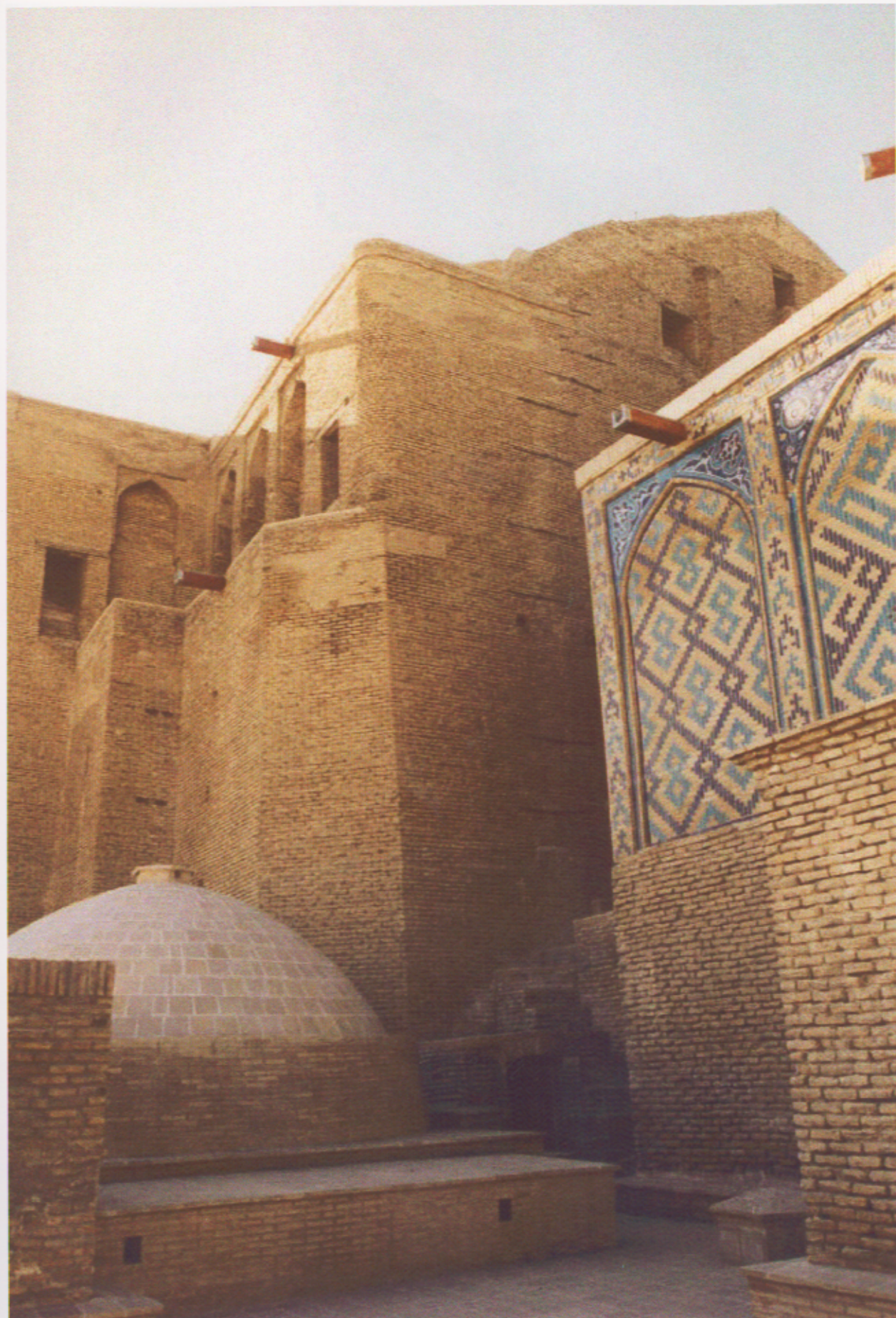
14. Rear side of portal, main drum and dome of well room
