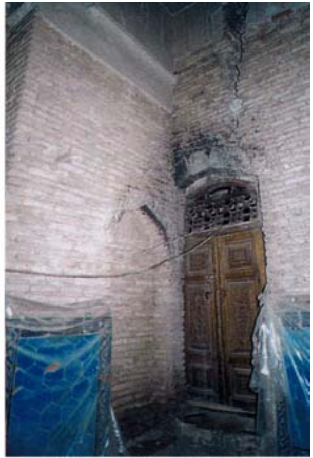
Masjid during restoration
