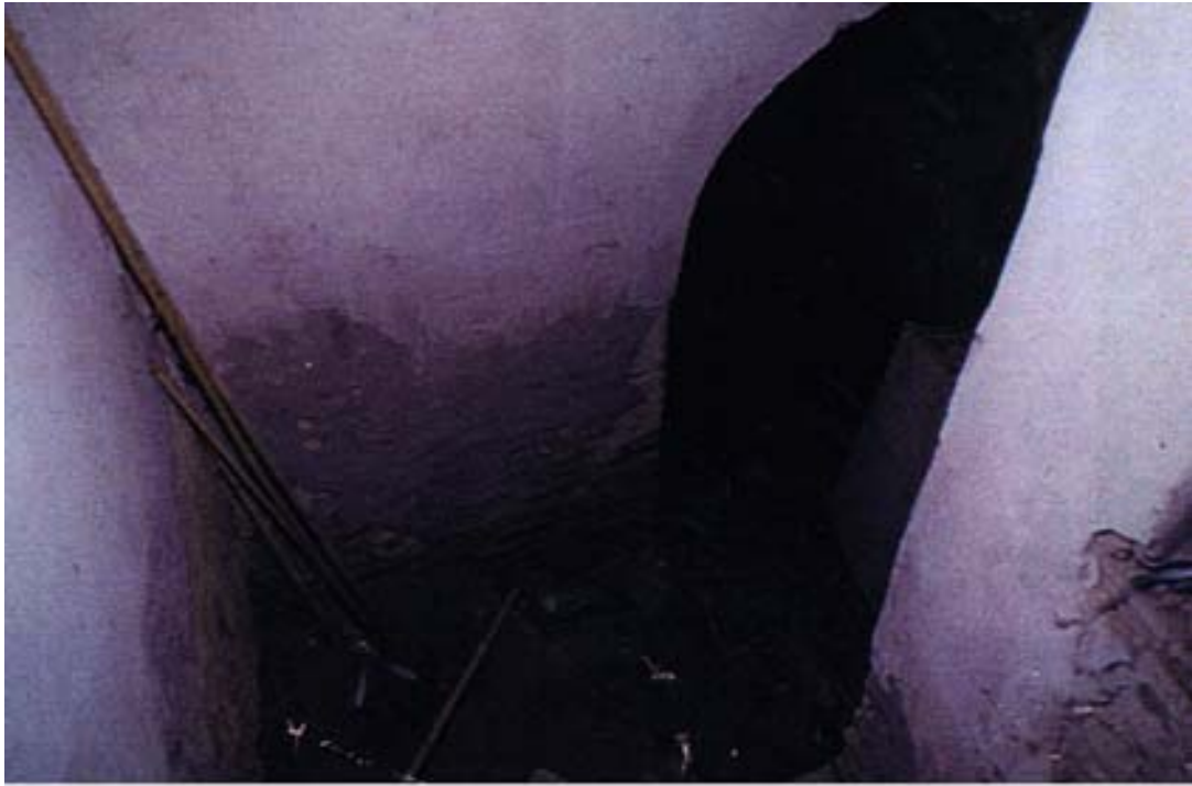
Stair before restoration
