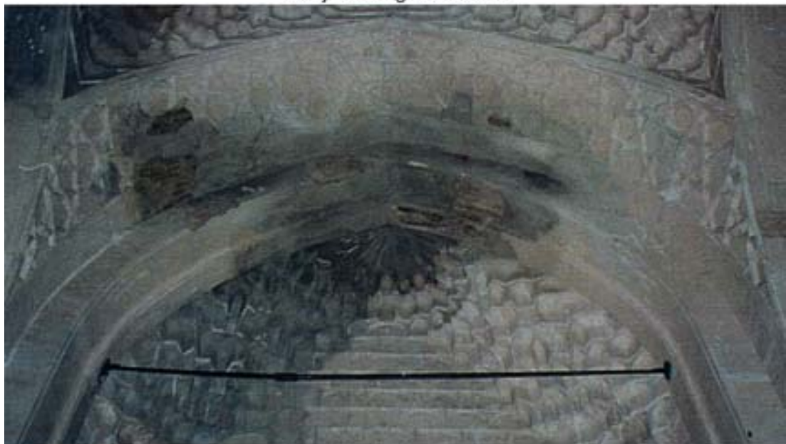
Masjid before restoration
