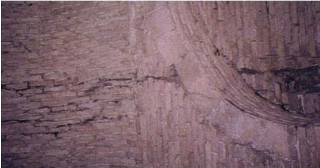
Corridor before restoration
