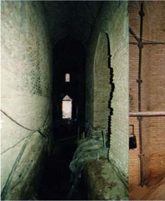
Corridor during restoration
