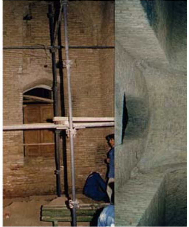
Corridor during restoration
