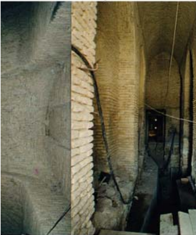
Corridor during restoration
