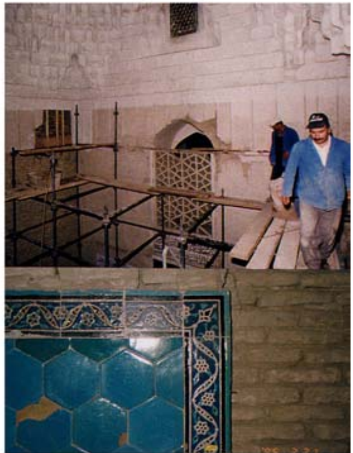
Masjid during restoration
