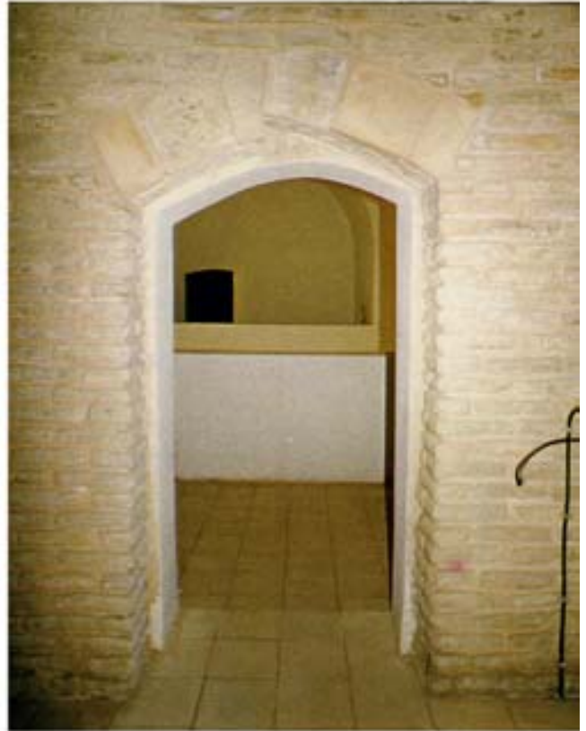
Room after restoration
