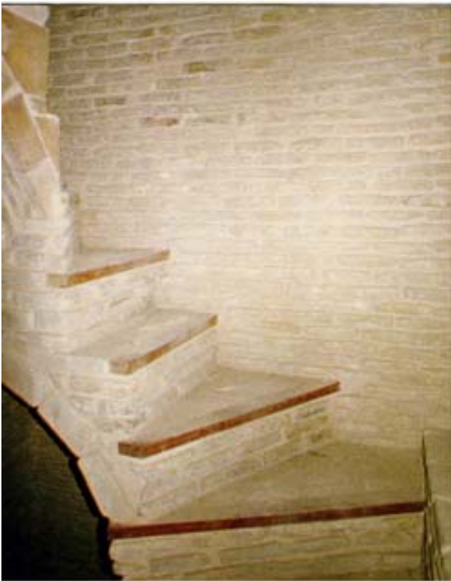
Stair after restoration
