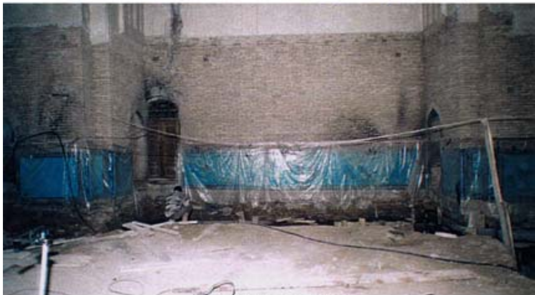
Masjid during restoration
