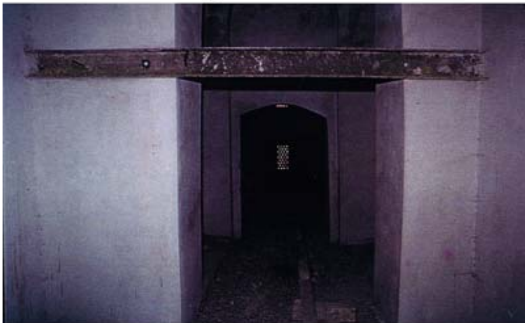
Corridor before restoration
