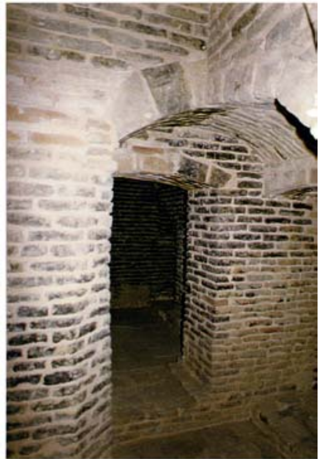
Corridor after restoration
