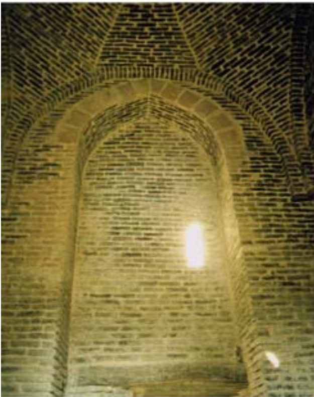
Room after restoration
