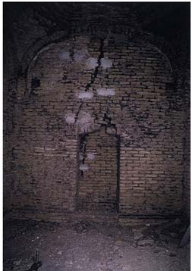
Room before restoration
